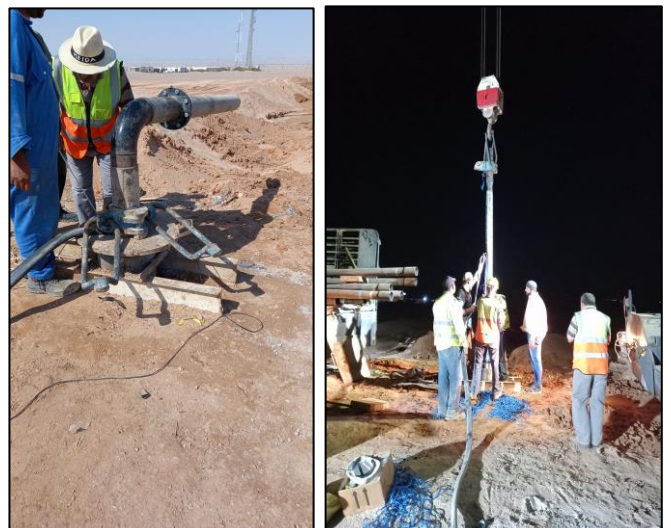
Figure 9: Cleaning the borehole with an air-jetting tool
